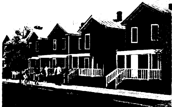
Figure 11 - Image of Restored Row Houses on Pasteur Street
